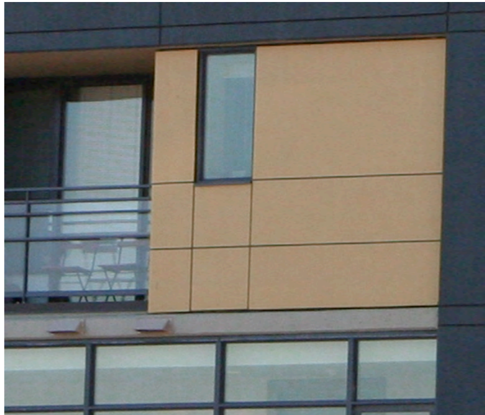
HARDIE BOARD PANEL ON EXTERIOR FACADE
